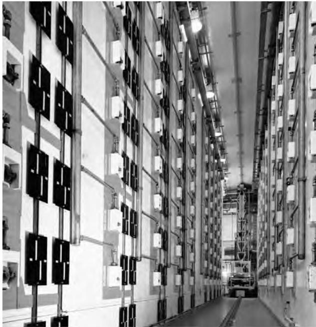
**Figure 6 UK Sellafield Product and Residue Store,** which became operational in 2011. Cans of plutonium are stored in separate lockers to protect against criticality accidents. *Source:* Sellafield Ltd.
